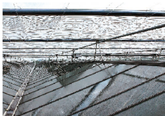
Using outdoor screens is one of the ways to filter NIR from entering the greenhouse.
